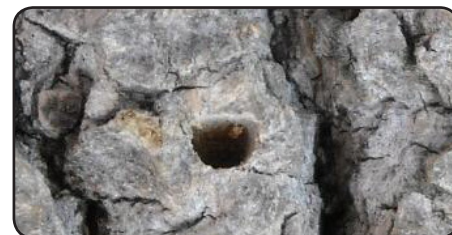
D-shaped borer exit hole.
