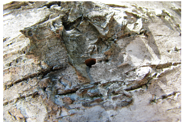
D-shaped exit hole.
